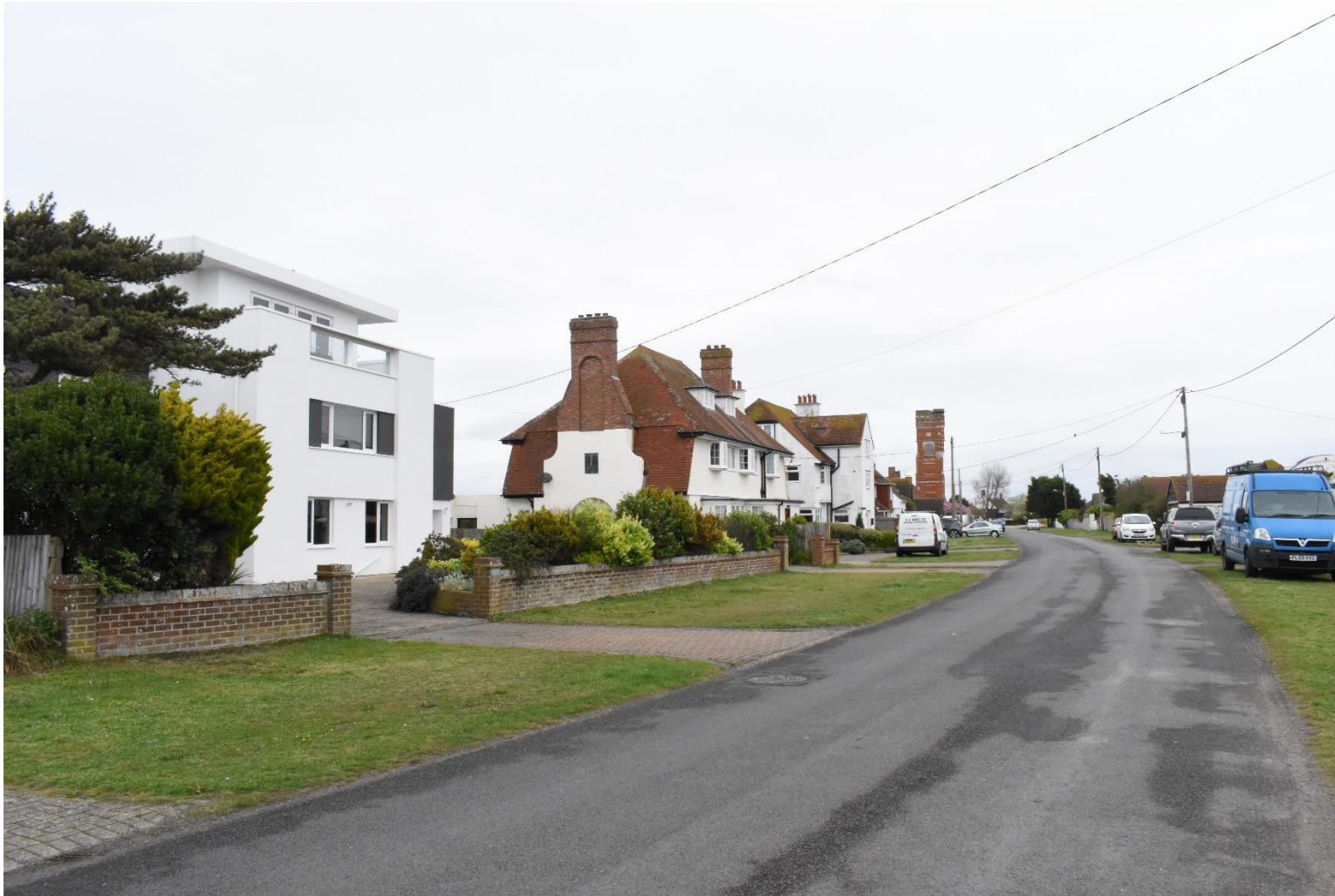
Plate 12: View Along Madeira Road towards the PDA (facing N)
